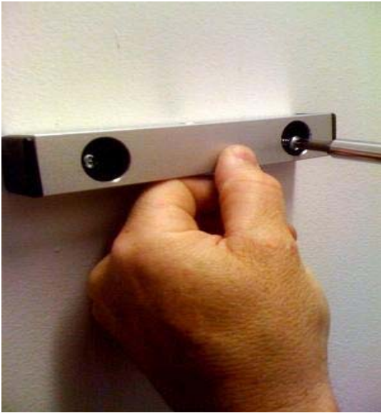
Fasten brace to the wall
