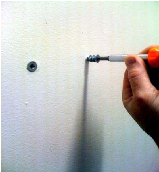
Screw self tapping fasteners (supplied) into the drywall
