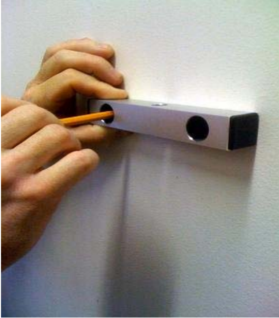
Mark the wall using the brace as a template
